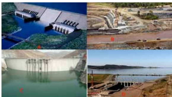
Figure 6: Examples of completed and under construction hydropower projects in Ethiopia: A. Design of GERD; B. GERD under construction; C. Tekeze and D. Beles Dams completed
